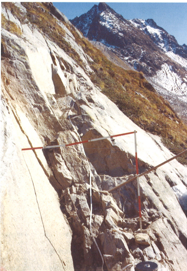
Fig. 67 from [9]: Dam no. 15 Cut groove in the smooth rock.
