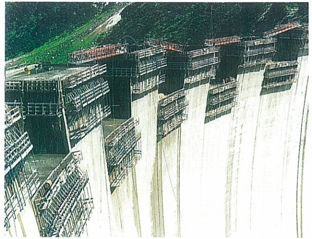
Figure 12 DOKA climbing formwork used at Kölnbrein and Zillergründl construction sites
