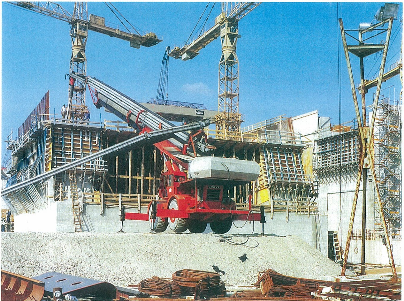
Figure 11 High speed conveyor belts on telescoping cranes pouring concrete at the construction site of the Melk power project on the Danube in 1980
