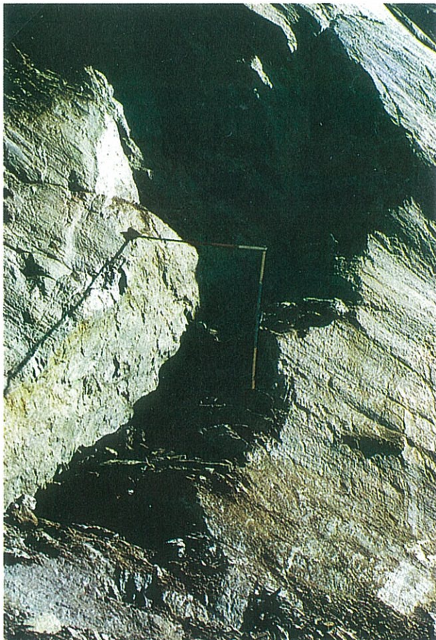
Figure 13 Finstertal dam – surface roughening for the bedrock
