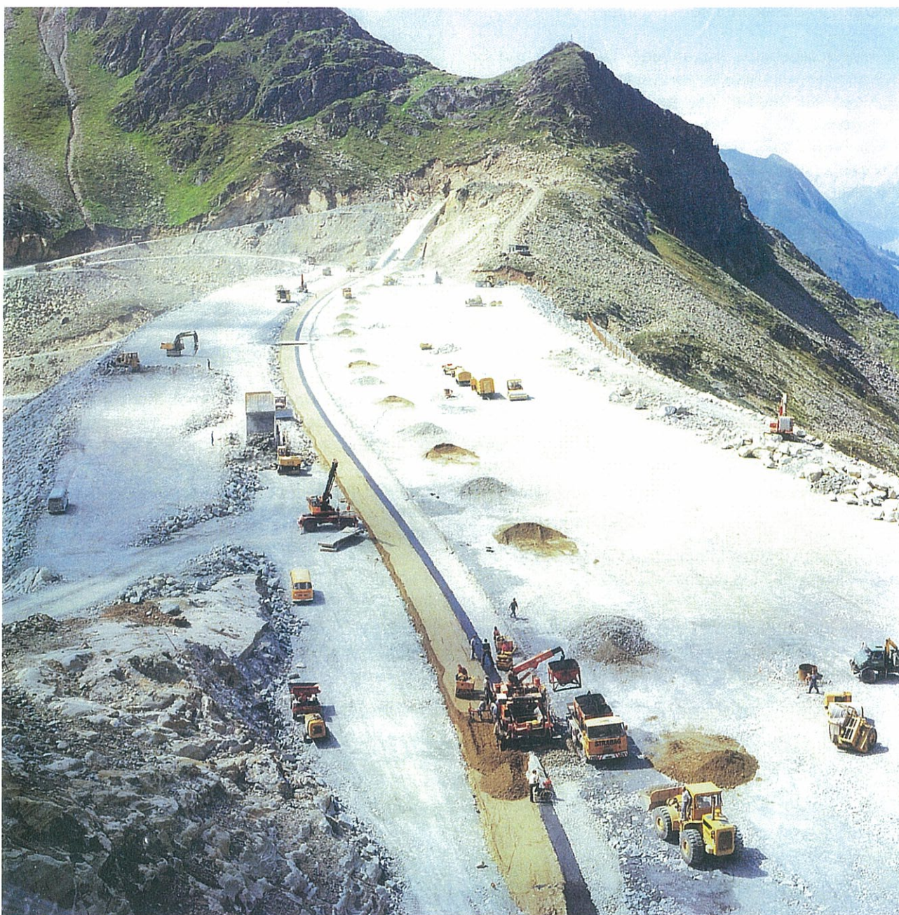
Figure 13 Placement of asphaltic-concrete core membrane at Finstertal embankment dam
