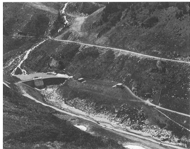
Fig. 49. Taschachbach stream intake (C) with concrete dam and frontal inlet
