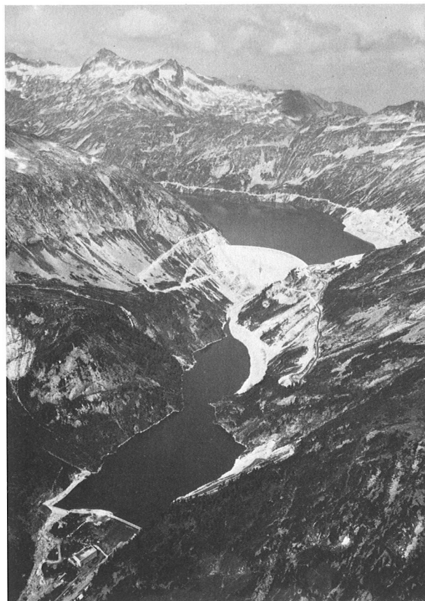
Fig. 40. Kölnbrein reservoir and arch dam (M1) as well as Galgenbichl intermediate reservoir and embankment dam (M2) with power station of Malta upper stage (M1)
