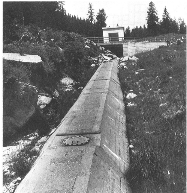
Fig. 54. Penstock of Wurten stage (K3) — Reinforced-concrete encased steel pipe without thrust blocks
