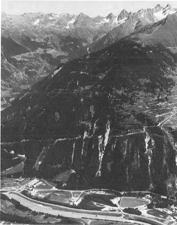
Fig. 51. Power shaft slope of Kaunertal scheme (C) with Prutz power station
