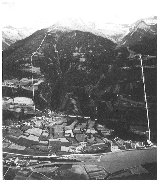
Fig. 37. Penstock of Reisseck stages (L1+L2) with Kolbnitz power station to the left as well as penstock from Malta main stage (M2) with Rottau power station and compensation reservoir of the Malta lower stage (M3) to the right
