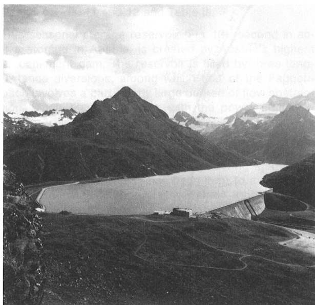
Fig. 9. Silvretta reservoir (A1) with Silvretta gravity dam and Biel embankment dam
