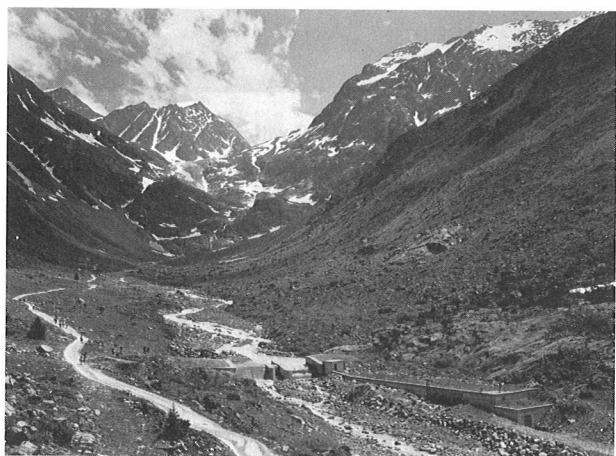
Fig. 48. Pitzbach stream intake (C) with horizontal coarse rack
