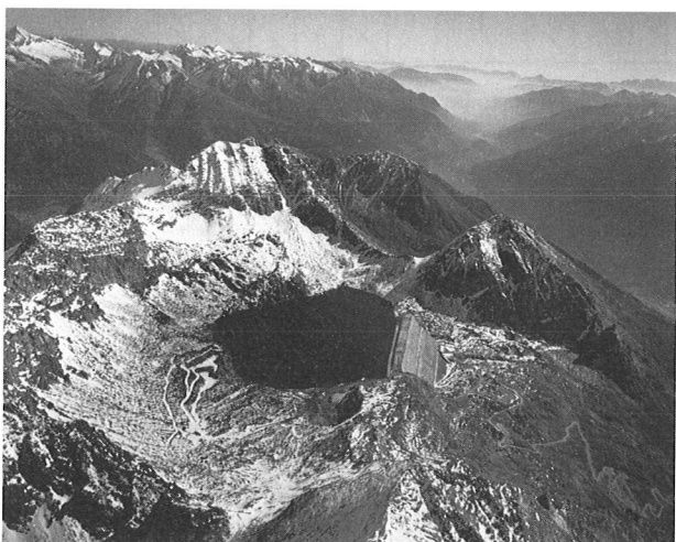
Fig. 47. Oscheniksee reservoir (K4) with rockfill dam with asphalt facing (released for publication by the BMFLV under ZI. 13080/254 — 1. 6./79)
